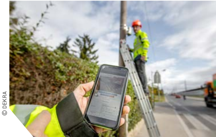
AIT transport researchers are installing the Mobility Observation Box, which collects high-resolution traffic data anonymously and on the move for up to ten days.
